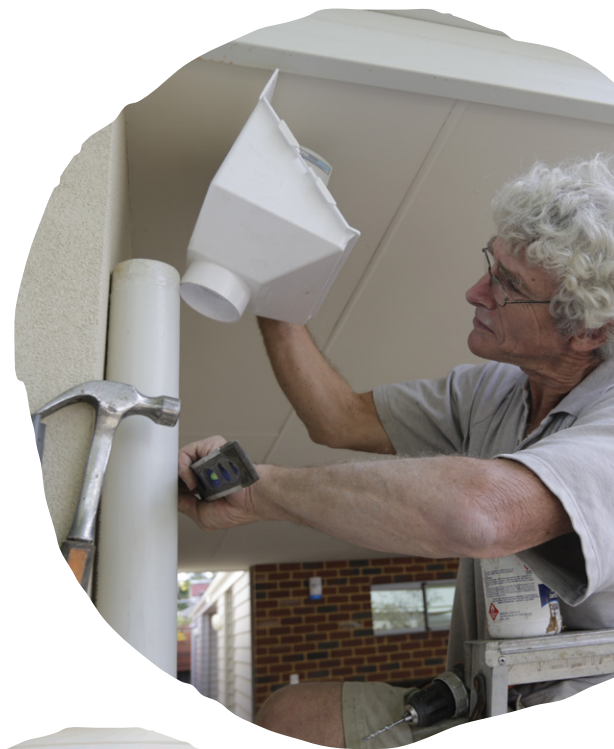
Installing rainheads to downpipes
