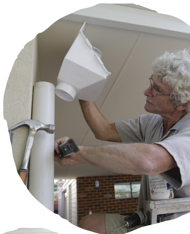
Installing rainheads to downpipes
