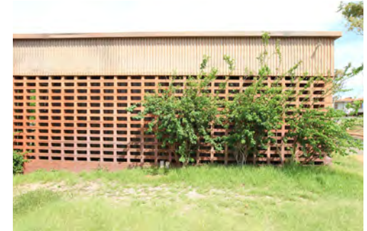
The old hospital in Port Hedland uses masonry breeze blocks to enable air flow and the brick conceals the dust accumulation on the exterior facade
