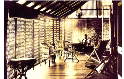
Original Broome covered verandah with permeable screens that blocks direct sun access, provides light and access to breeze
