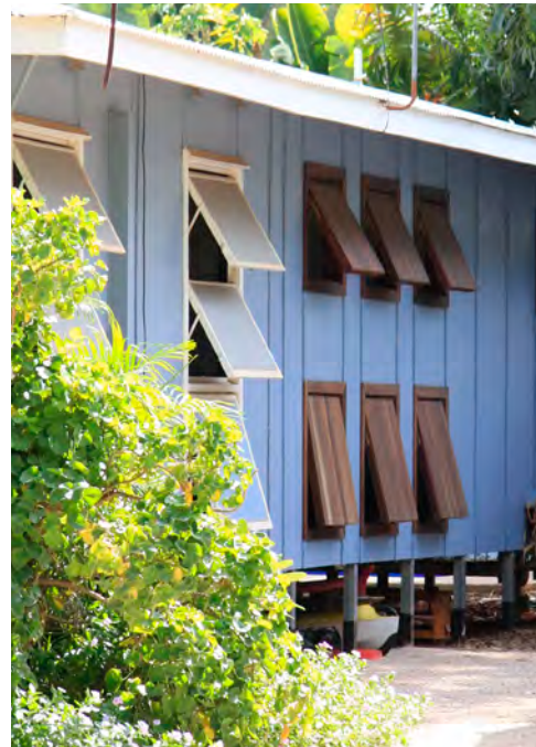
Solid panel awnings over non-glazed openings show effective high and low level ventilation - Broome
