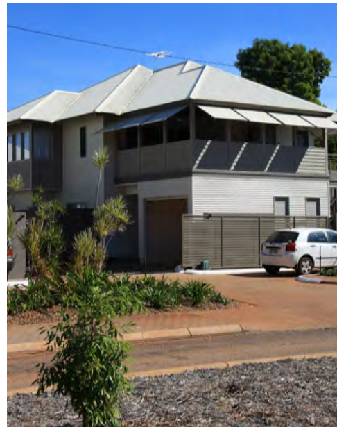
First floor verandah with shutters for shading and ventilation and cyclone security - Broome
