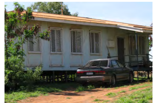
Lightweight steel frame on stilts construction in Onslow Dampier
