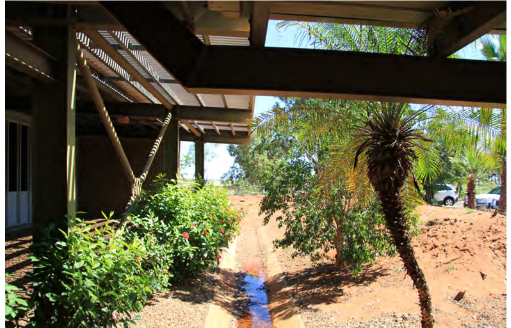
In ground gutters channel stormwater away from the building at the Pilbara TAFE campus - South Hedland
