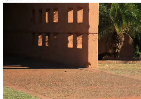
Rammed earth construction using local pindan soil - Port Hedland (left) and Newman
