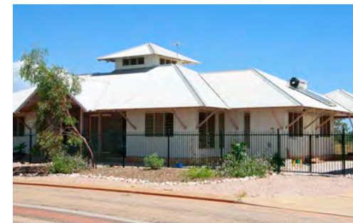
This house has a combination of elements that would reduce electrical usage - a solar hot water unit and operable windows to release hot air from the interior
