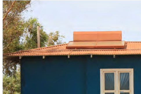
Take advantage of the high number of sunshine hours in the Pilbara and use solar energy or hot water systems. Note dust build up on roof
