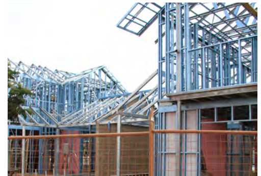
Lightweight steel frame with concrete blockwork. Townhouse development - Newman
