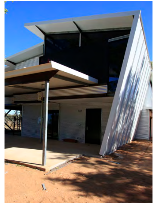
Wing wall incorporated into wide eaves - Kununarra
