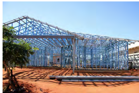
Steel framed construction perform well in cyclonic conditions. Any weakness is usually in the connections
