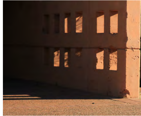
Rammed earth construction using local pindan soil, South Hedland
