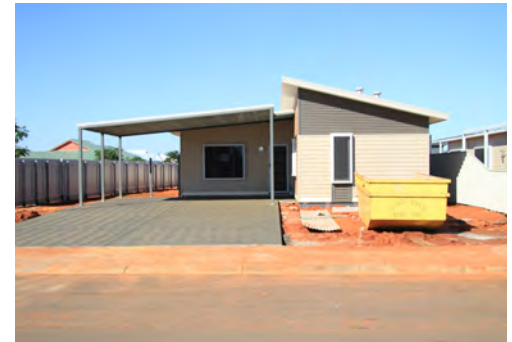
Lightweight construction in South Hedland. Steel frame on slab, house
