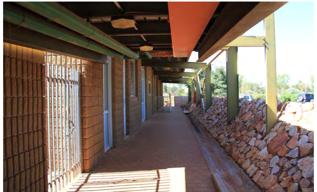
Local stone berm walls at Pilbara TAFE, South Hedland Campus. Note the shaded blockwork and perimeter drainage at the base of the retaining wall
