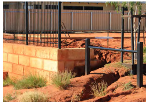
Heavy rainfall will quickly erode recently completed developments that have not had time to for vegetation to establish - South Hedland
