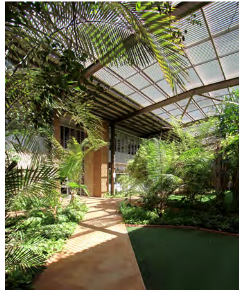
Large courtyards incorporating shading devices and vegetation are supplemented with wall mounted fans to maintain a cool temperature at Pilbara TAFE
