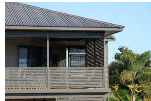
A contemporary sun protected verandah with breeze permeable composite aluminium screening to allow for breeze flow in Port Hedland
