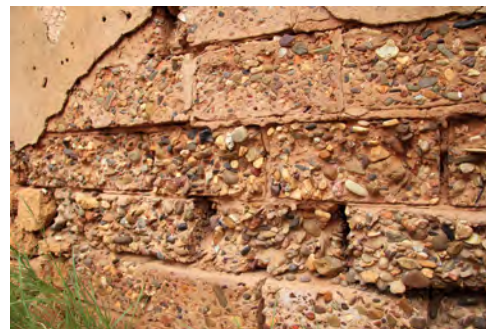
Locally sourced materials used to make clay, riverstone and gravel bricks - Old Onslow
