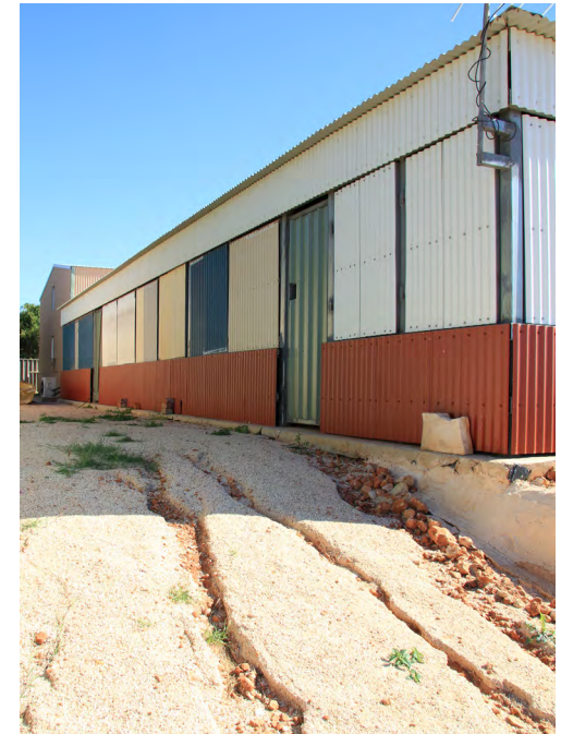
Erosion as a result of not addressing roof drainage - Exmouth
