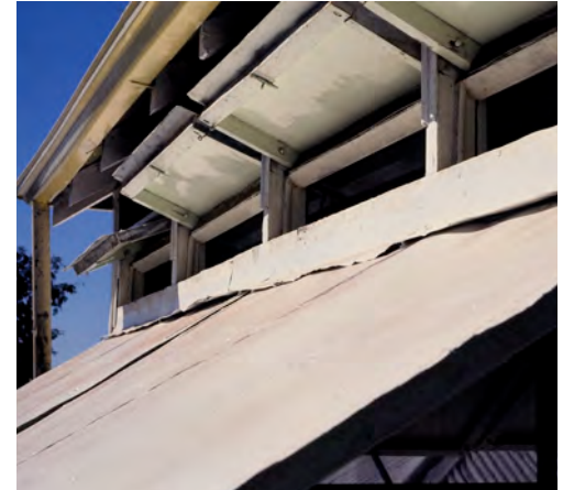
Openings under the eaves allow hot air to escape. These openings have solid panel awnings to block late afternoon sun - Broome
