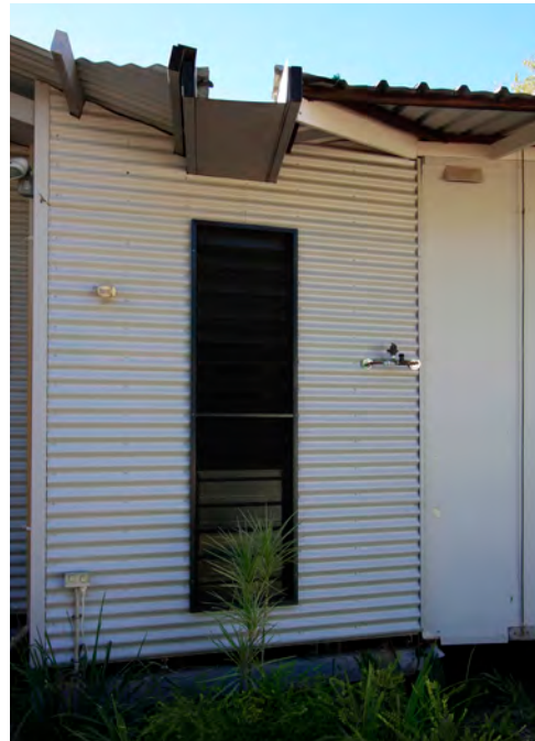
Box gutter sized for heavy downpours of rain. Water flows straight into garden - Kununurra
